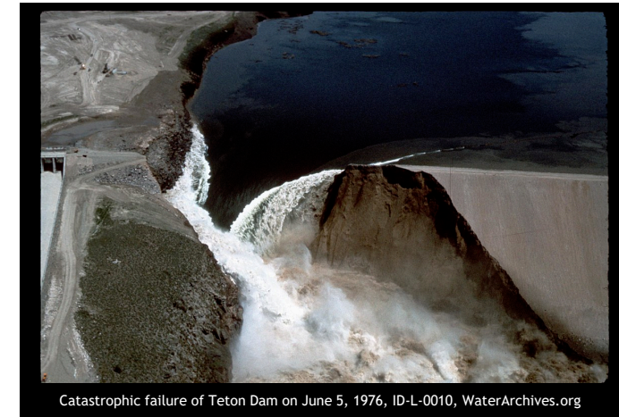
Catastrophic failure of Teton Dam on June 5, 1976, ID-L-0010, WaterArchives.org
